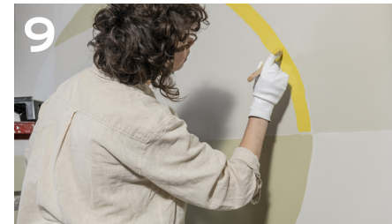
9 Make sure to use a paint brush to cut in.
