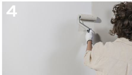
4 Paint your first colour with a roller. This acts as a base layer.
